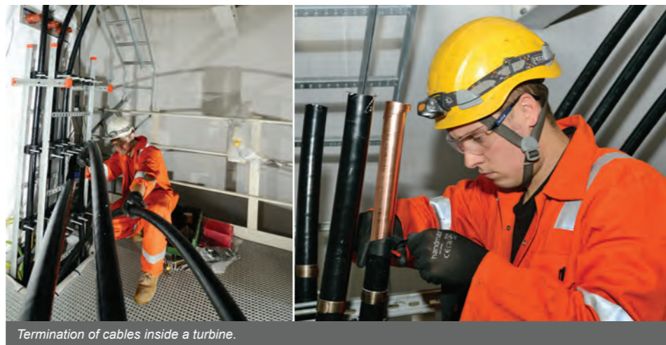
Termination of cables inside a turbine.
