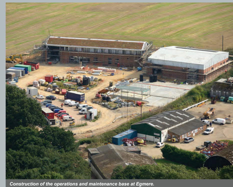
Construction of the operations and maintenance base at Egmere.
